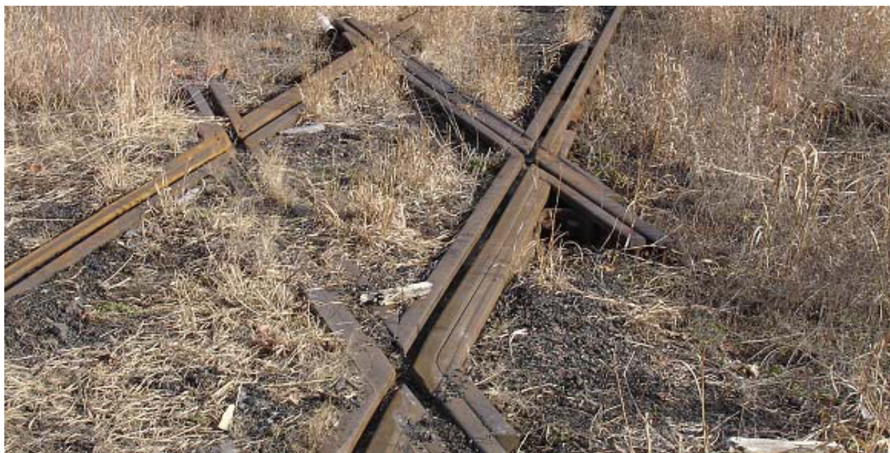
Near the roundhouse remains is a lone track diamond. Although the crossing track appears to run into equipment, beyond that equipment is the bridge to the Lehigh Valley Railroad's former Bowman's Creek Branch.
