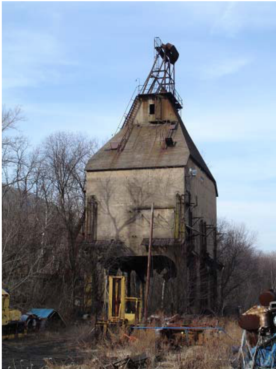
North of the roundhouse and diesel shop stands one of Coxton Yard's former coaling towers. To state that it's immense is an understatement—note the stairs climbing to its apex. The tower contains at a minimum seven tender distribution chutes, which were fed by the sloped mechanism to the rear (left) of the tower.
